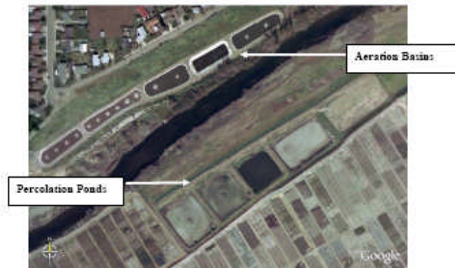
Figure 9 City of Waterford Existing Wastewater Treatment System Ponds
