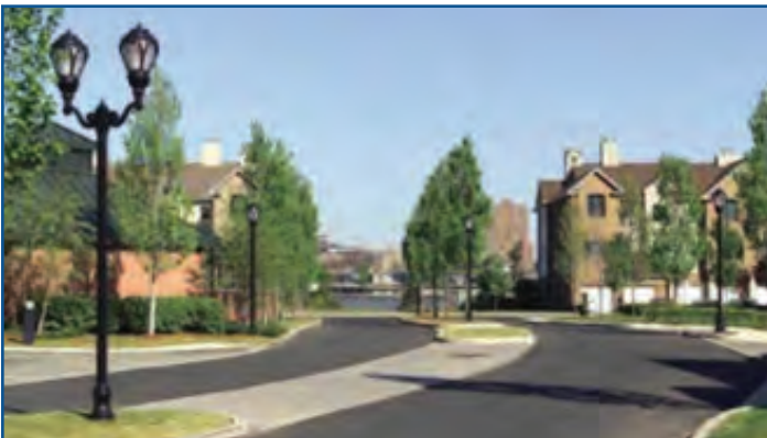
Double-headed decorative lighting along collector street
